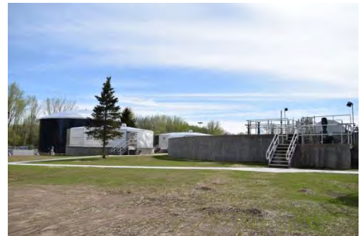
Clintonville Wastewater Treatment Facility
