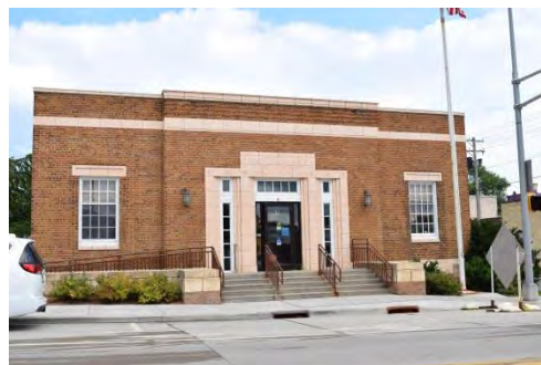
Clintonville Post Office
