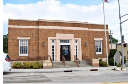
Clintonville Post Office
