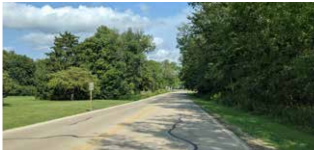
Existing conditions on Fire Lane 12
